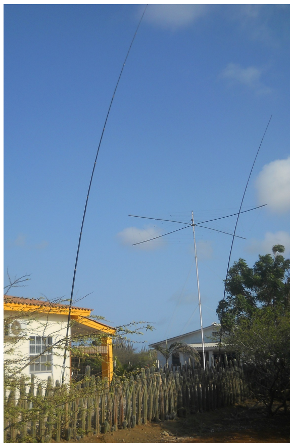
Antennas at PJ4DX: 40m phased vertical array (working again now!) and Spiderbeam at 30ft / 9m high.
