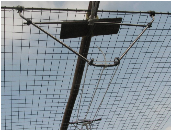
Figure 6: tensioning of the screen and radiator..
